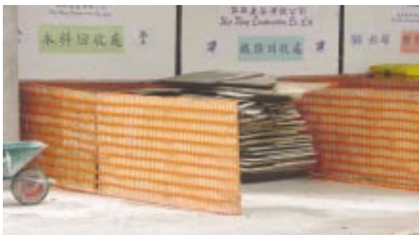
Waste sorting for recovery during construction at The Orchards
