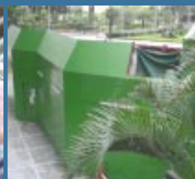
Specially designed hoarding for minimising noise impact at Three Pacific Place
