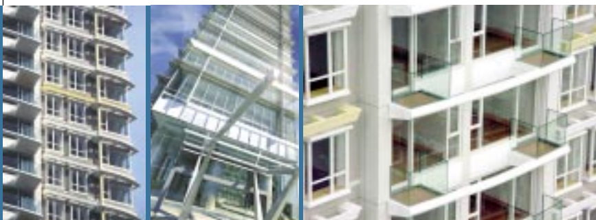
The Orchards external sunshades Three Pacific Place fins and façade The Orchards balconies
