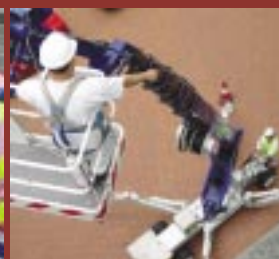
Close communication during use of mobile plant
