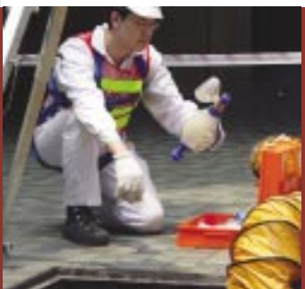
Confined space work
