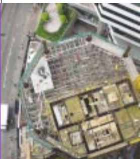
Formwork and pre-cast beams
