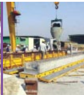
Pre-fabrication yard off-site
