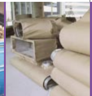
Pre-fabricated duct work
