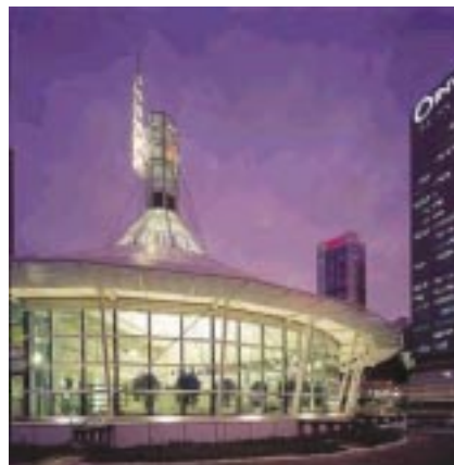
Exterior of the INTEGER pavilion
