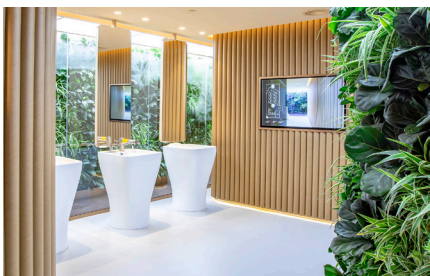
The interior walls are made of 100% recycled and recyclable paper tubes
