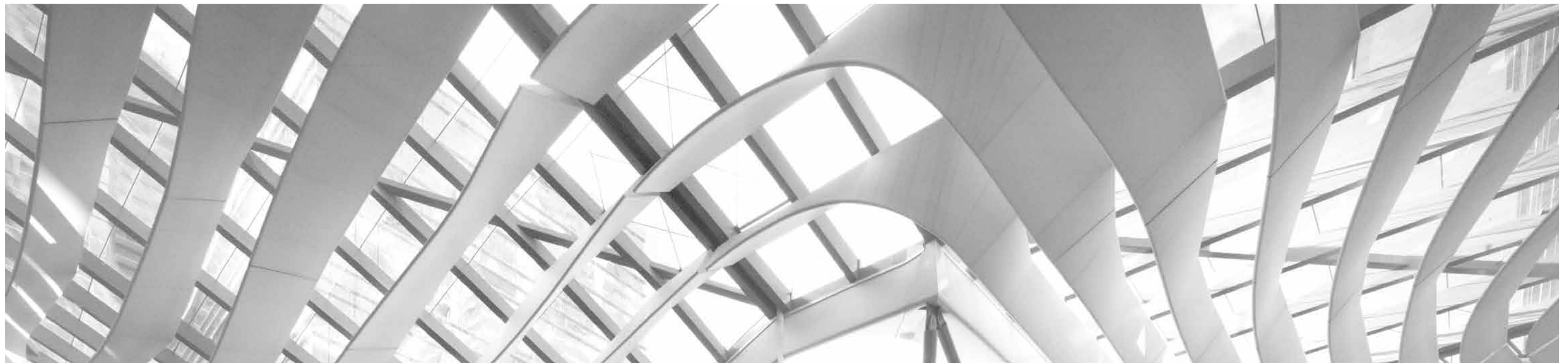
A 100,000 sq ft faceted canopy of steel and glass undulates between the mall, hotel, offices and residential towers
