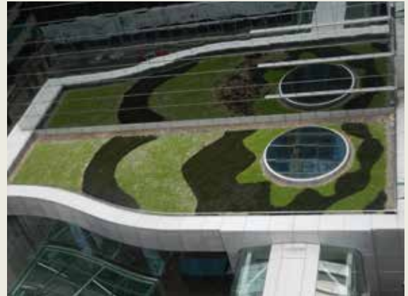
Oxford House New Green Roof
