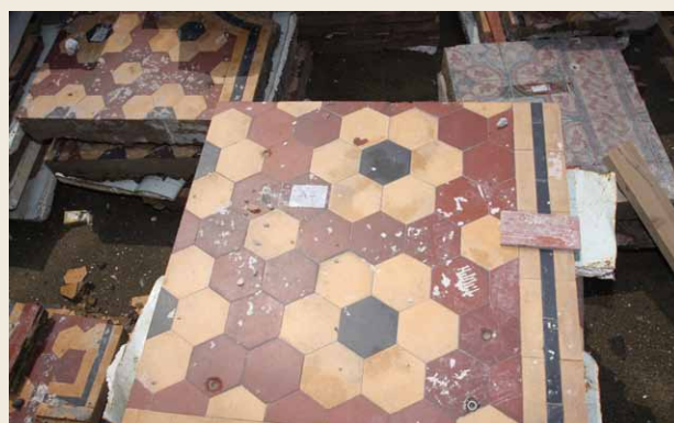
Tiles were removed and labelled during relocation work
