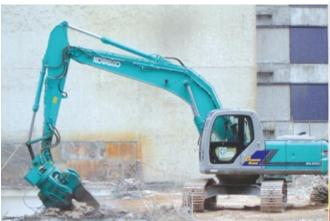
Hydraulic crushers reduce noise during construction.
